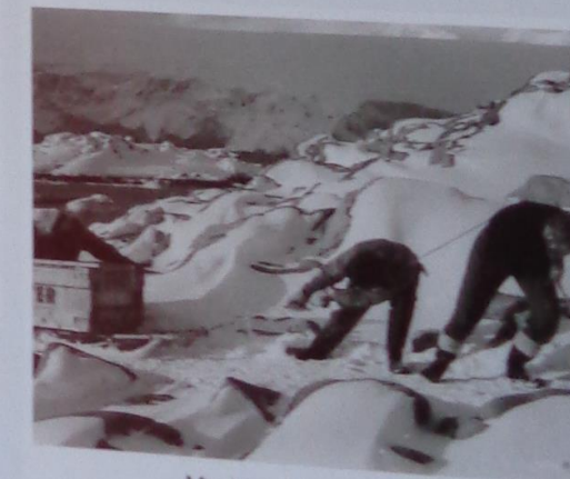
Moving generator parts
