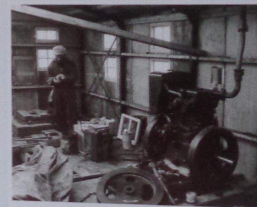
Installing diesel generators
