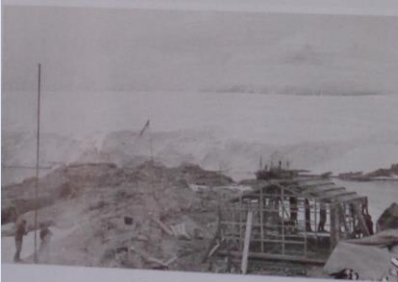
Building the hut
